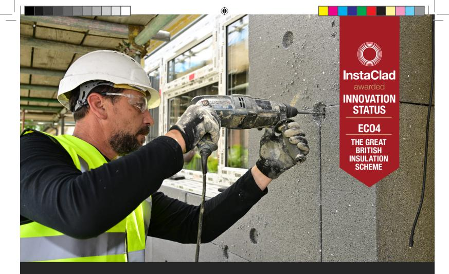
We installed InstaGroup's leading External Wall insulation system InstaClad Robust on the walls, and Stomix StxTherm Robust below the DPC.
